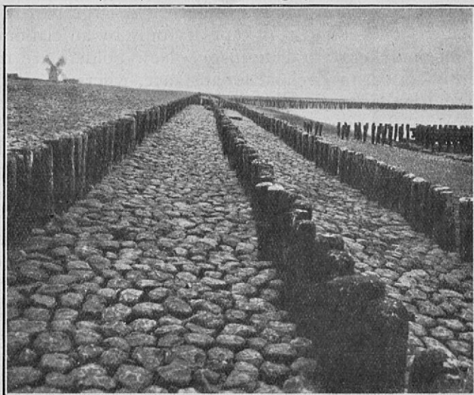
Wooden Piles of the famous Dutch Dyke of Westkapelle
