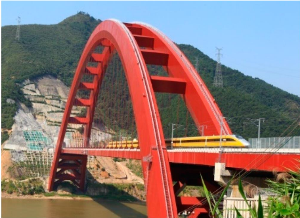
Figure 11. Wind barriers installed on the Xijiang Bridge in China (Zou et al. 2019).
