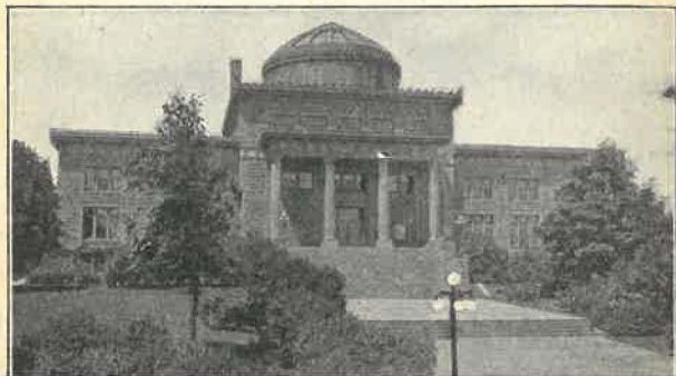
Marquette County Courthouse. Scene of the Roosevelt-Newett libel suit in which Roosevelt was awarded six cents.
