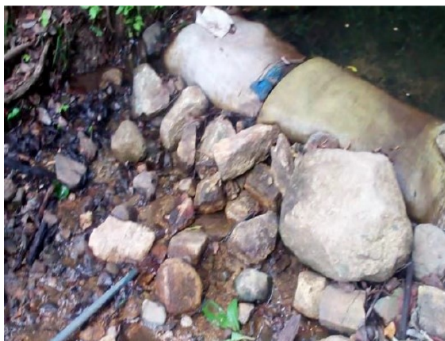
Figure 20, Rudimentary dam built with sandbags (Chikuhwa, 2021)
