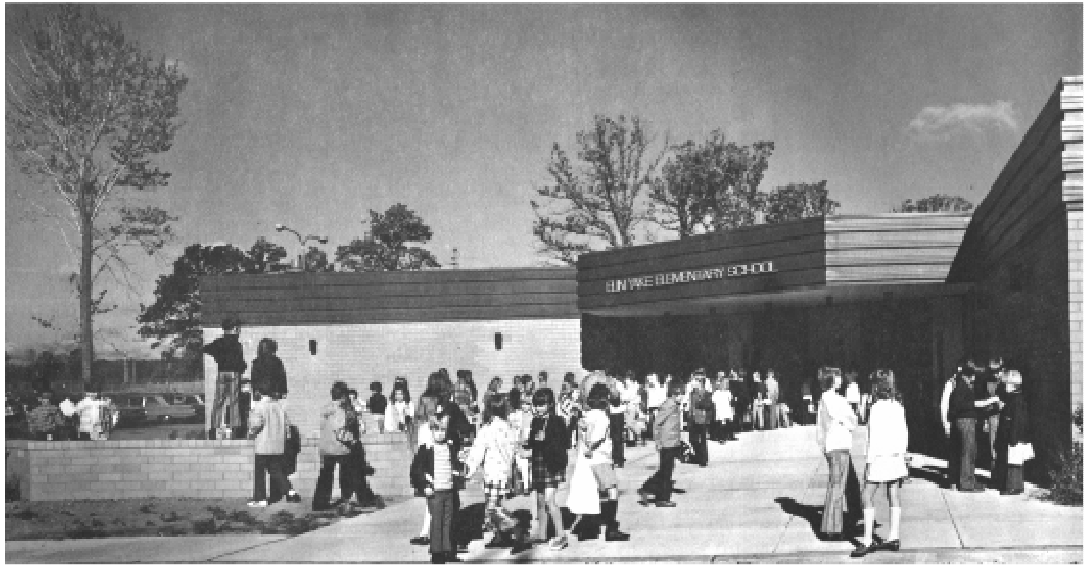
Illustration 32. The Elin Yake Elementary school represents the second and partly the third phases of Kainlauri's school architecture (1971).
