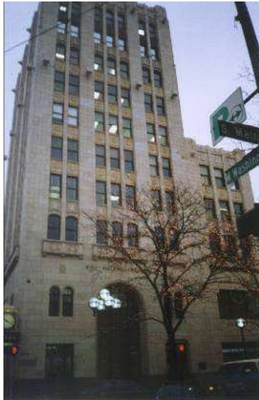
Illustration 26. Fry & Kasurin, The First National Bank Building in Ann Arbor was finished in 1929.
