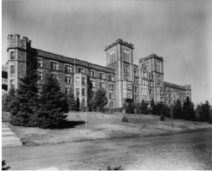
Illustration 19. F. German and A. W. Lignell, Duluth Tower Hall, College of St. Scholastica 1906-1908
