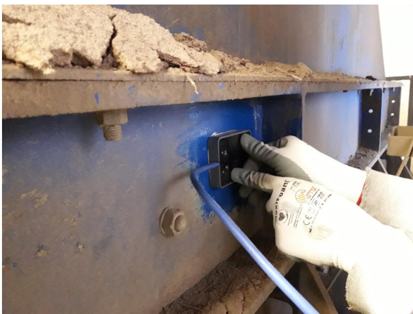
Figure 4. Vibration sensor installation
