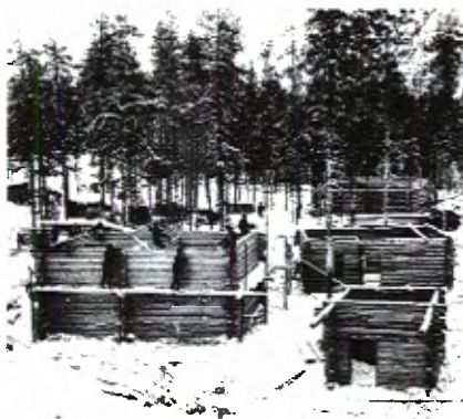
121. The "house factory" of Division 3 near Uhtua in 1942 produced more than 100 Aseveli houses. Photo SRM.
