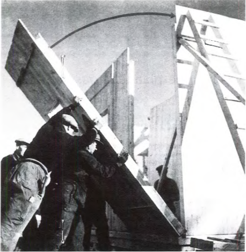
92. Workmen raising a standardized single-family house, the A-talo , designed by Alvar Aalto and published in the leaflet advertising A-talo . A-talo - tulevaisuuden talo .
