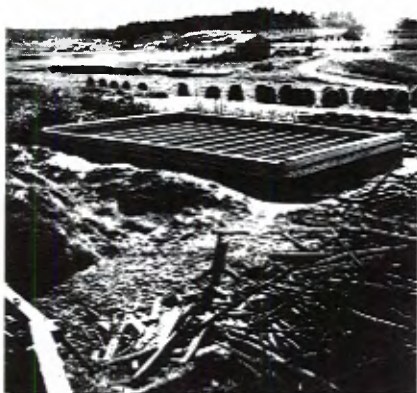
122. The foundations of an Aseveli house. Photo SRM.
