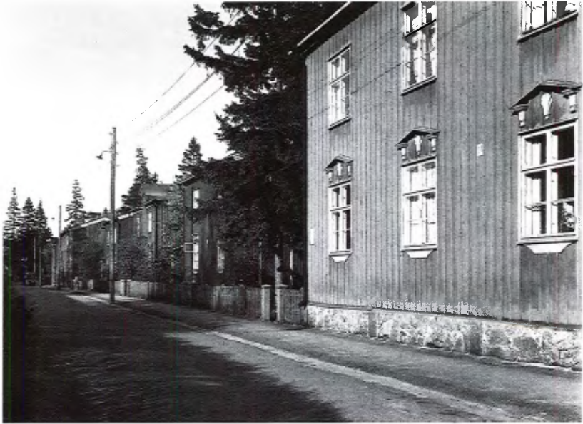
64. Puu-Käpylä, Tapiolantie. Photo Heikki Havas, beginning of the 1960s. HKM.
