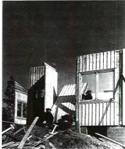
2. Construction of "Swedish houses" in Pirkkola, Helsinki, 1940. Published in Arkkitehti 2/1941, p. 24. Photo SRM.
