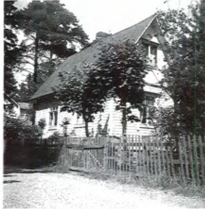
9. Single-family house in Tapanila, Helsinki. Photo Eino Leino. HKM.
