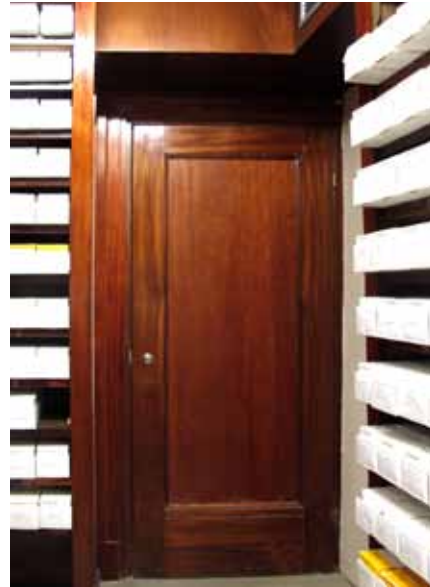
Ovi 2: Mahonkinen umpipeilinen kehysovi.
