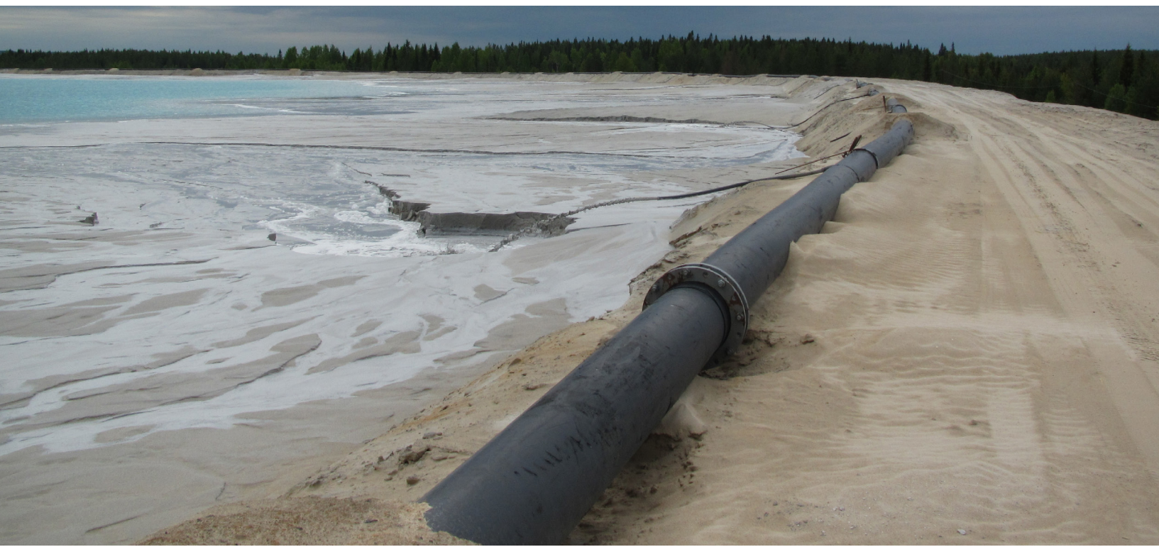
Taililings dam raised using tailings material, 2012 (Timo Regina)
