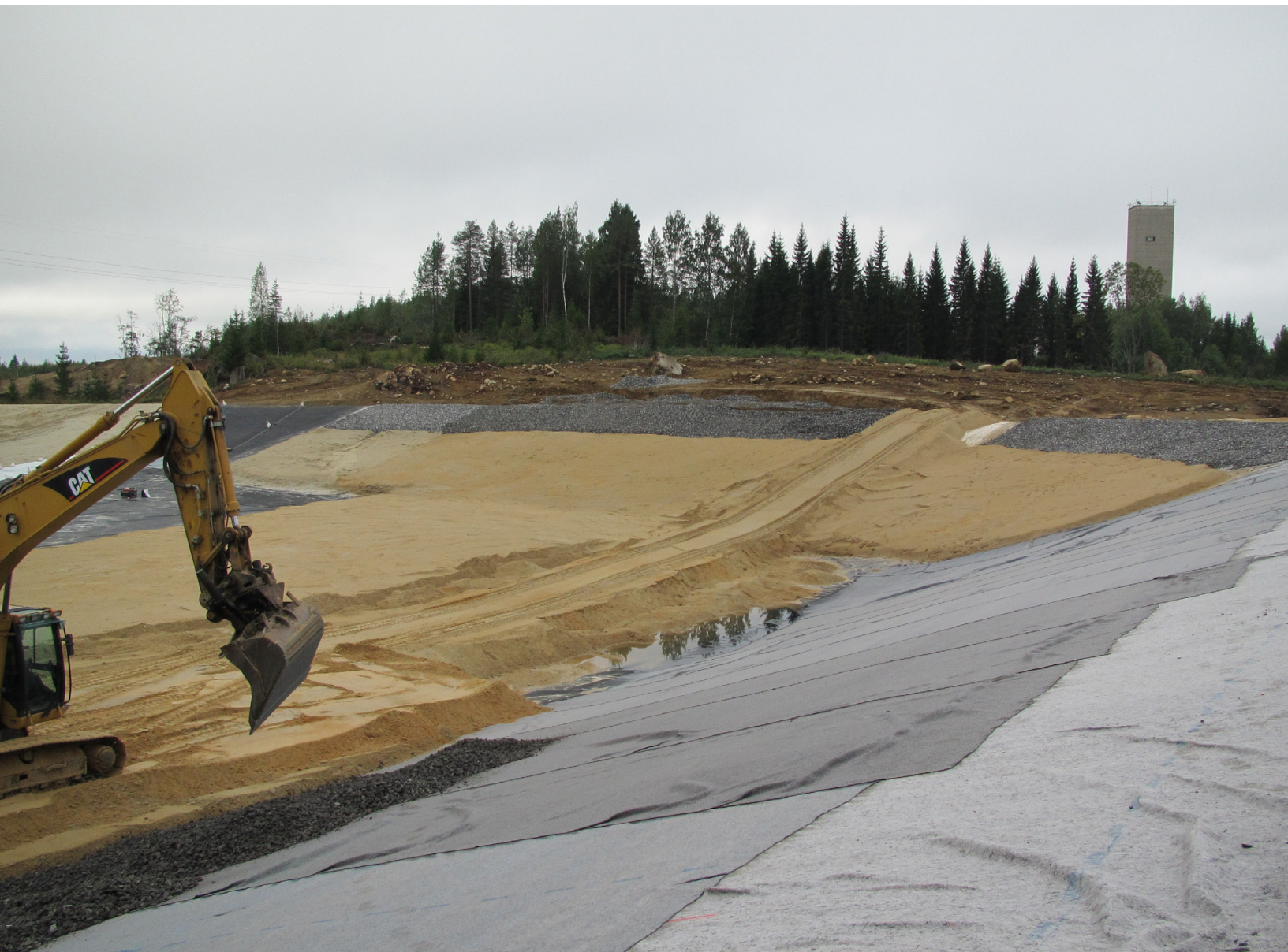
Tailings dam under construction in Luikonlahti, Kaavi, 2011 (Timo Regina)
