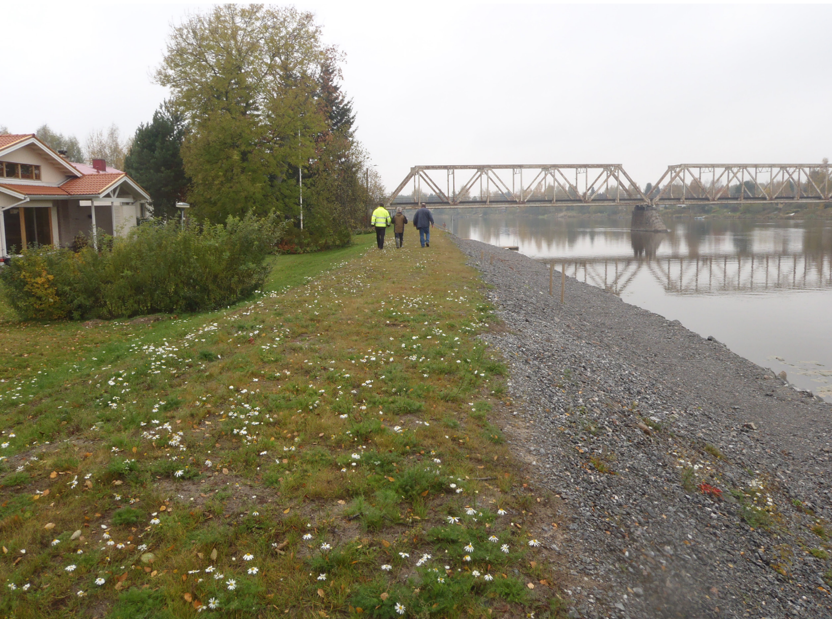
Repaired flood embankment, Pori, 2010 (Milla Torkkel)
