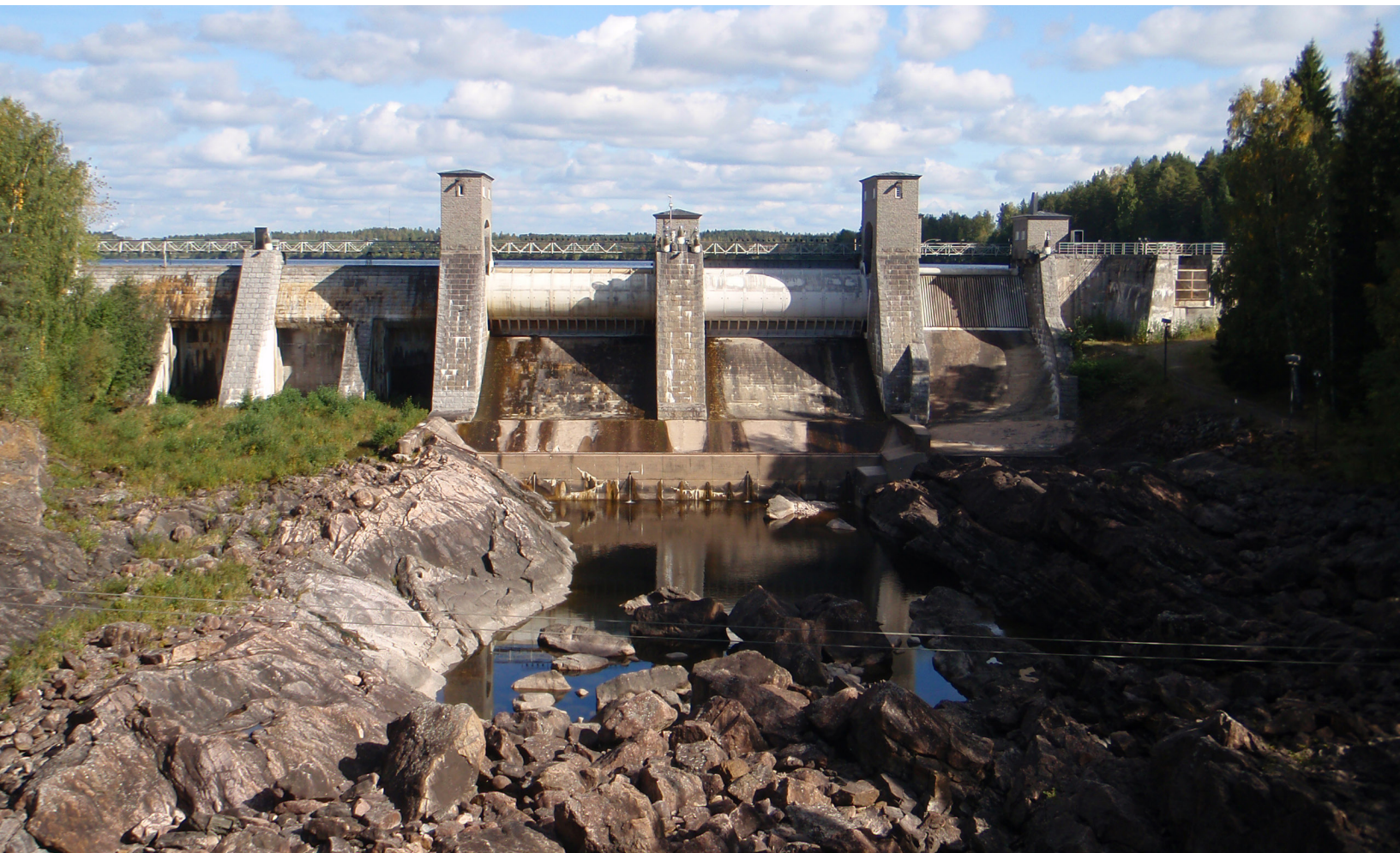
Imatrankoski regulating dam, 2010 (Milla Torkkel)
