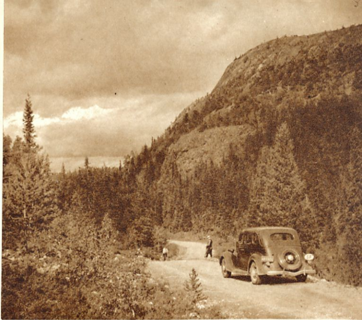
Motor roads have been built through the wilds of Kuusamo.
