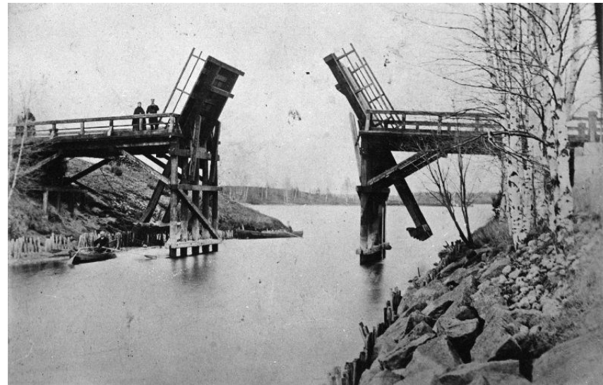
Bascule Bridge. Tampere Historical Museums
