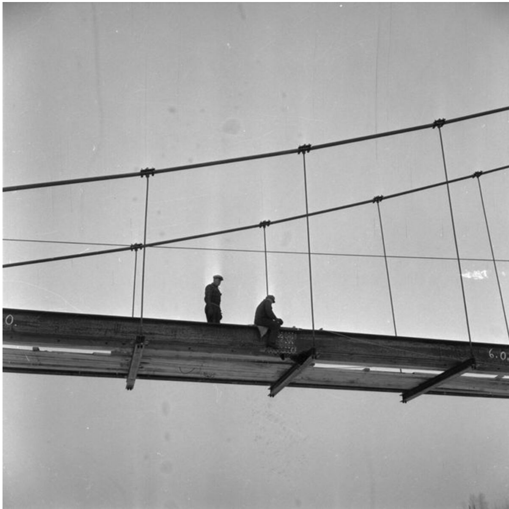
Kiettare bridge. Seppälä, Raimo, photographer. Satakunta Museum.
