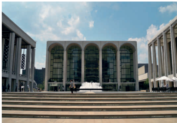
BILD II.26. Flera arkitekter under Wallace K. Harrisons ledning. Lincoln Center , https://en.wikipedia.org/wiki/Lincoln_Center_for_the_Performing_Arts#/media/File:Lincoln_Center_by_Matthew_Bisanz.JPG . 27.3.2017.
