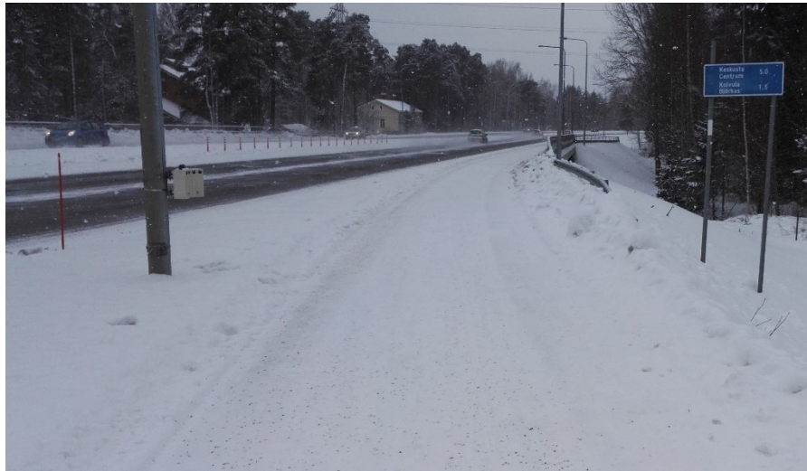
Figure 37 Weather and road conditions on Wednesday 7.2.2018 13:59, also showing the second location of the northern ViaCount -device (ViaCount (north) 2) (Peltonen, 2018).
