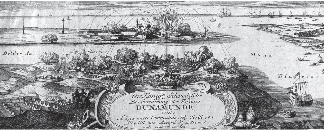
Picture 4.22 The picture above, of the Swedish siege of the fortress in 1701, provides a good idea of both the fortress and the location. It was a modern bastion fortress, sited on the outer tip of an island. The expanses of the Baltic Sea are seen in the background. (Source: Die Königl Schwedische Bombardirung der Festung Dunamunde , nr 1701:22, Volume 14 Omslag 1701–1704, Förteckning 426 Historiska planscher 1520–1904, Krigsarkivet.) (Detail)
