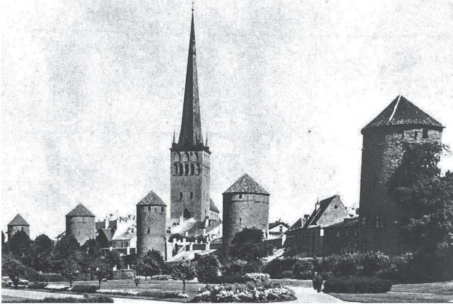
Picture 4.28 The photograph above shows the medieval western part of the Reval defenses. The flat ground in front of the walls created an example of high attacker's local accessibility, in other words, it was not difficult to reach the walls. The photograph was probably taken in the 1940s. (Source: Armin Tuulse, Borgar i Västerlandet (Stockholm 1952), Plate ["plansch"] 55. Photographer unknown.)
