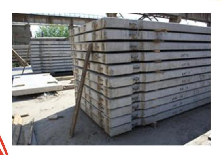
The strength of PAG slabs is provided for by the use of pre-stressed reinforcement in the longitudinal direction, however no prestressing is provided for in the transverse direction.
