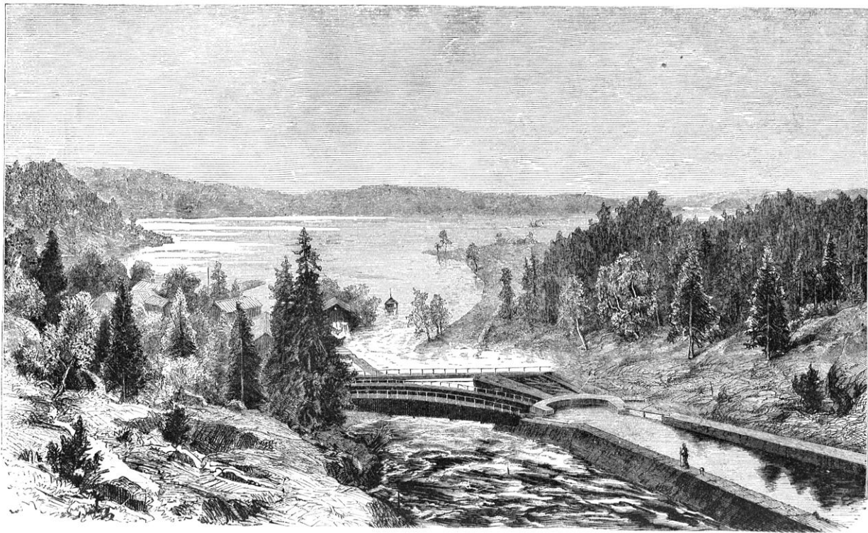
VIEW ON DALSLANDS CANAL.
