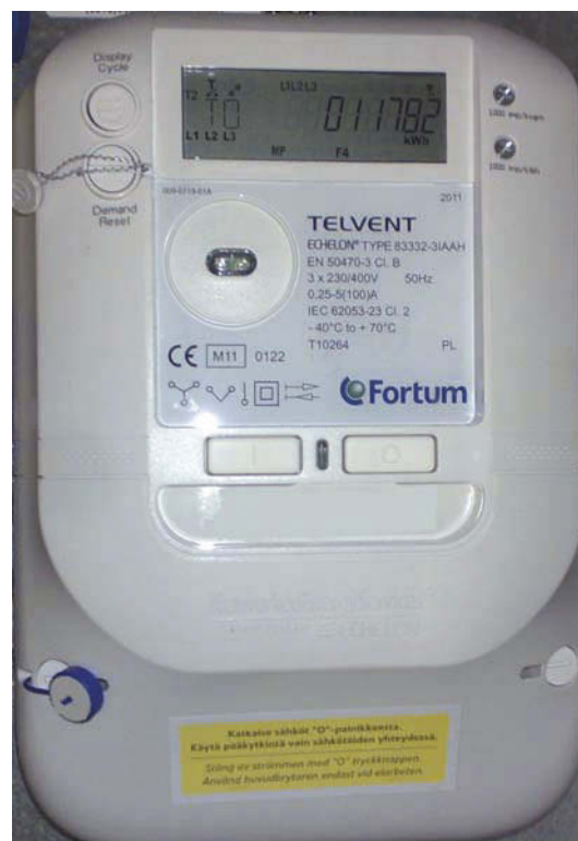
Figure 6. Smart meter, Photograph: Heinäaro, Kimmo
