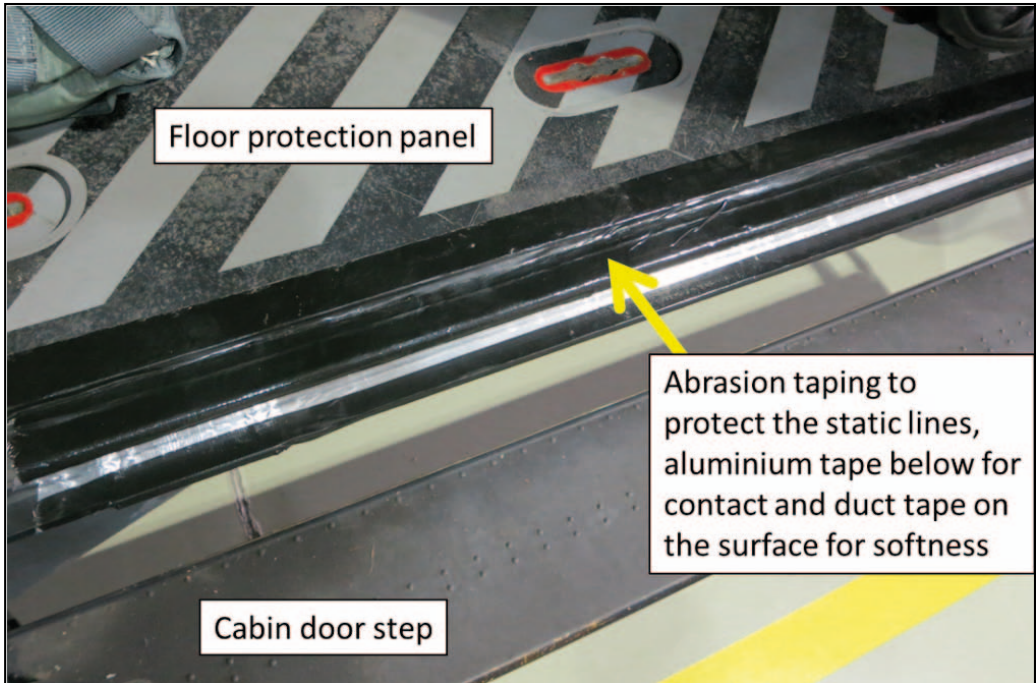
Figure 13. The right side cabin boarding step with Patria’s floor protection panels and the abrasion taping installed. The aluminium or “high-speed” tape was of the following type: 3M, width 50 mm, P/N 425 BWB 1194–38. The duct tape type was Würth 50 mm x 50 m SUPERBLACK, P/N 1985 505 05
