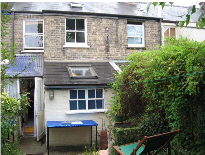
28. Hale Street, Cambridge, July 2007: "a decrepit terraced cottage in the Castle Hill area of the city".
