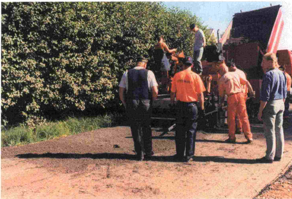
Figure 11: Compacting on a crushed stone layer
