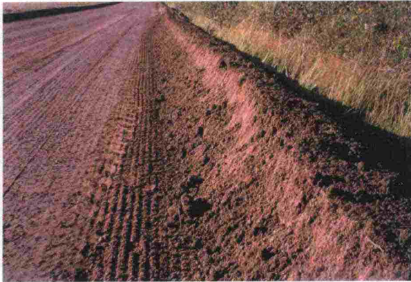
Figure 4a: Preparing for construction
