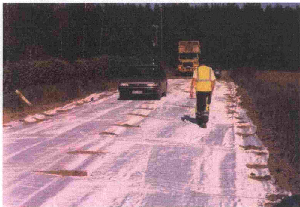
Figure 6: Geotextile spread on an embankment
