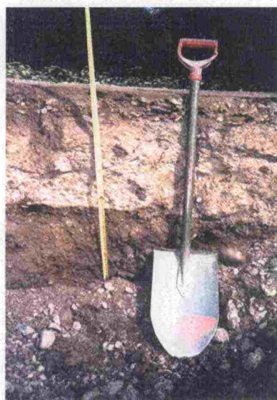
Figure 7: Stabilized structure; a mix of gypsum and lime
