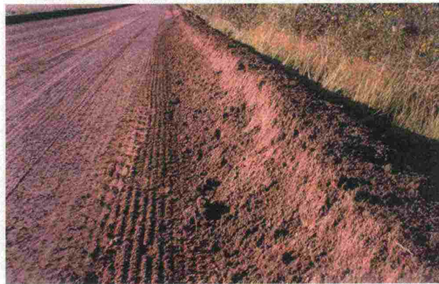
Figure 2a: Preparing for construction
