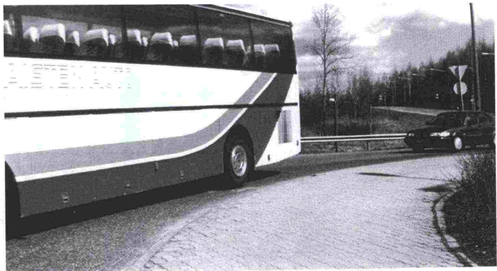
Figure 17: Truck apron structure at the roundabout of Hämeenlinna.
