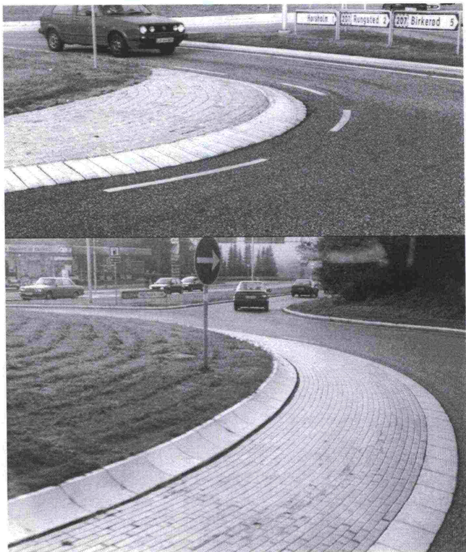
Figure 23: Truck apron structure at the Hämeenkyrö roundabout.
