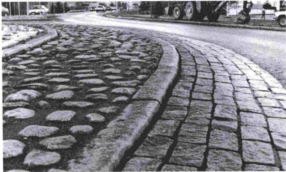
Figure 23: Truck apron structure at the Hämeenkyrö roundabout.
