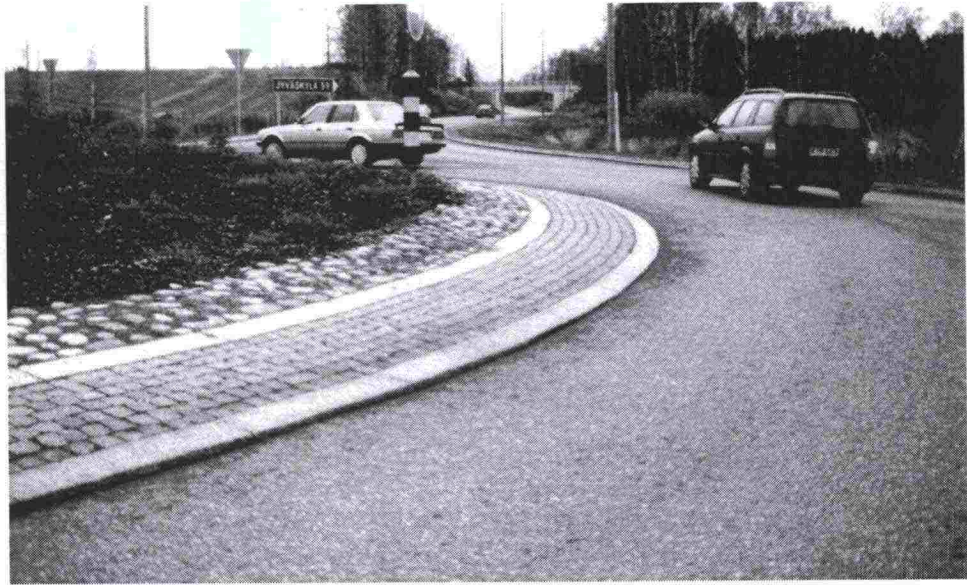
Figure 21: The truck apron structure at the Jämsä roundabout.
