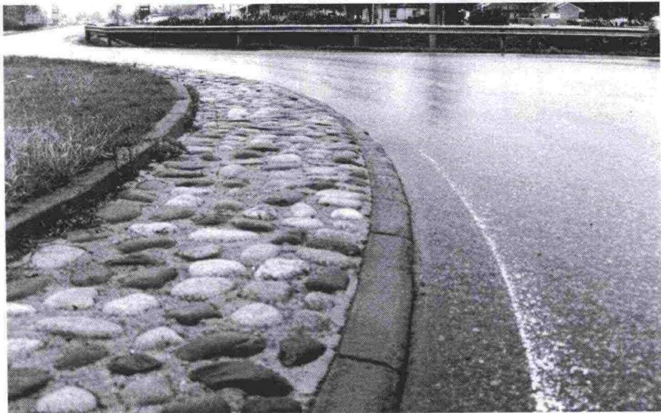
Figure 21: The truck apron structure at the Jämsä roundabout.
