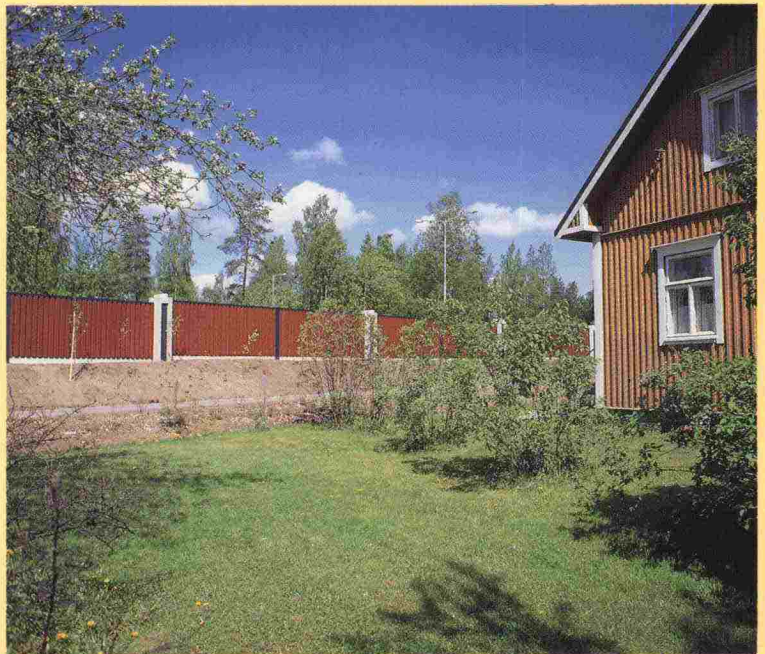
Noise barrier by the Tuusula motorway, as seen by residents in 1994.
