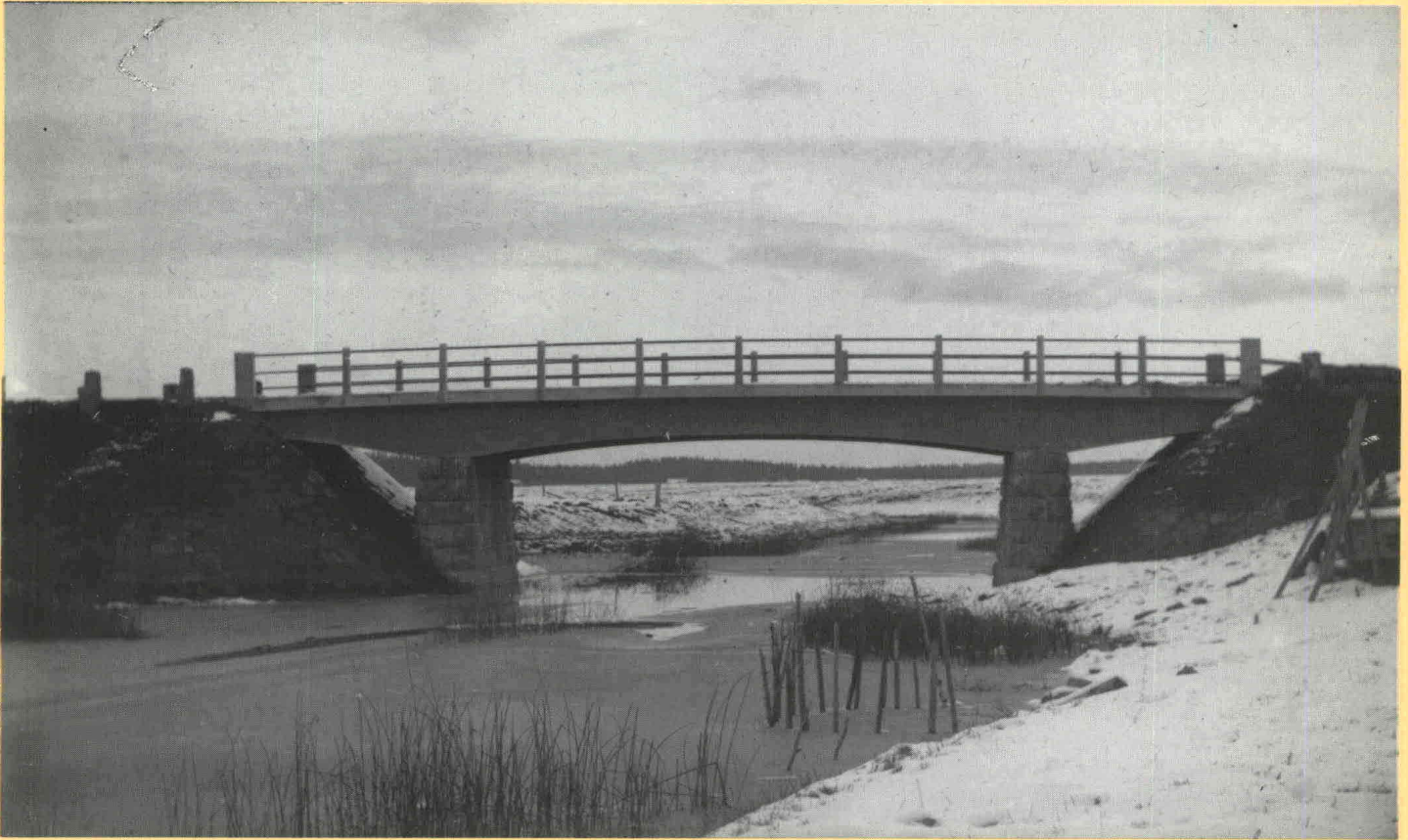
A cantilever bridge of reinforced concrete in Elimäki in 1926. New and strong.
