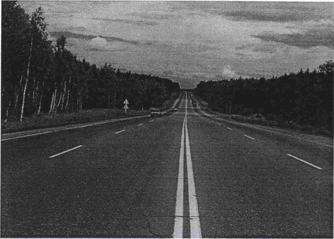
Figure 1. Some main road sections are in good condition.
