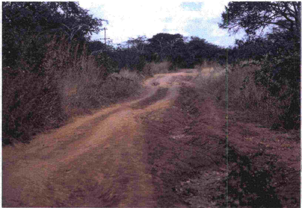
Figure 1. A rural road in a poor condition in Zambia. The place in the district road D154 near Lusaka where the red clay was taken for the laboratory tests (Chapter 4.).
