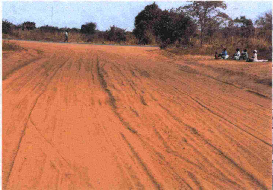
Figure. Class 1. The shape of the road may have changed. There are many corrugations, ruts or potholes. The surface is not solid and there may be very soft places. Very dusty.
