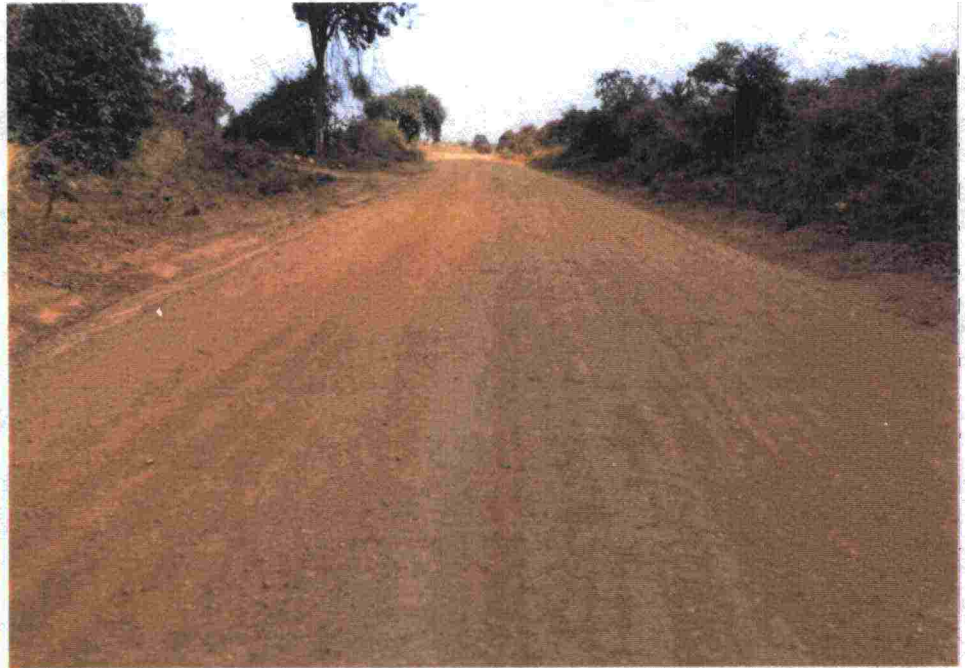
Figure. Class 3. The shape of the road is quite good and the surface of the road is quite even. About half of the surface is solid. There are some corrugations, ruts or potholes. Dusty.
